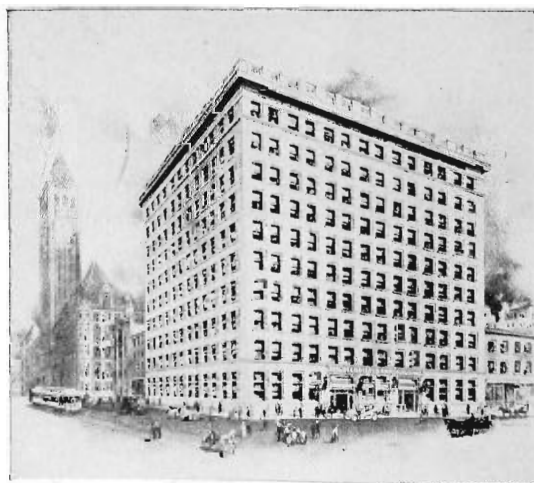
SECURITY BANK BUILDING.
